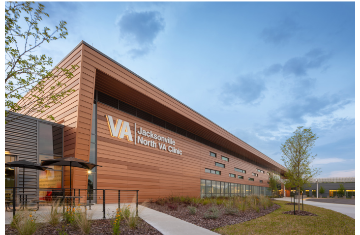
Jacksonville North VA Clinic & Domiciliary Two Green Globes Certification
